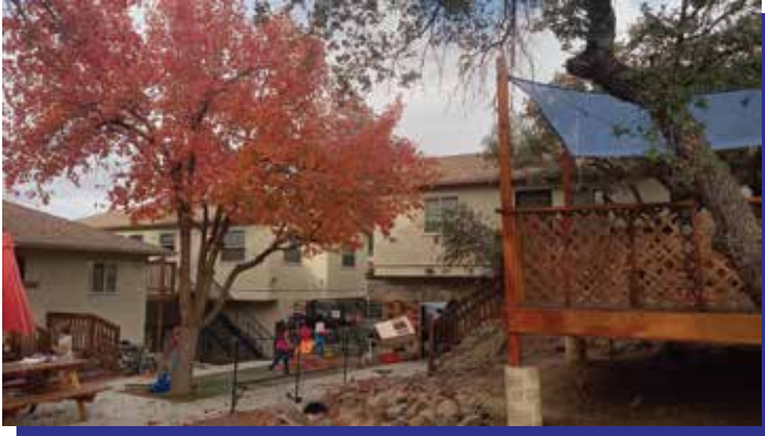
Prescott NINE UNIT COMPLEX
